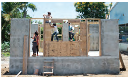
The 2019 Design/Build project: one-room schoolhouse in Loiza, Puerto Rico
